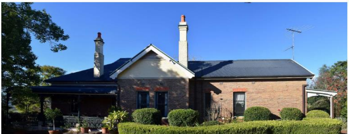
Figure 15 Koorana Homestead Complex
