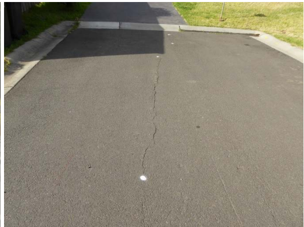
Tahmoor House Court
