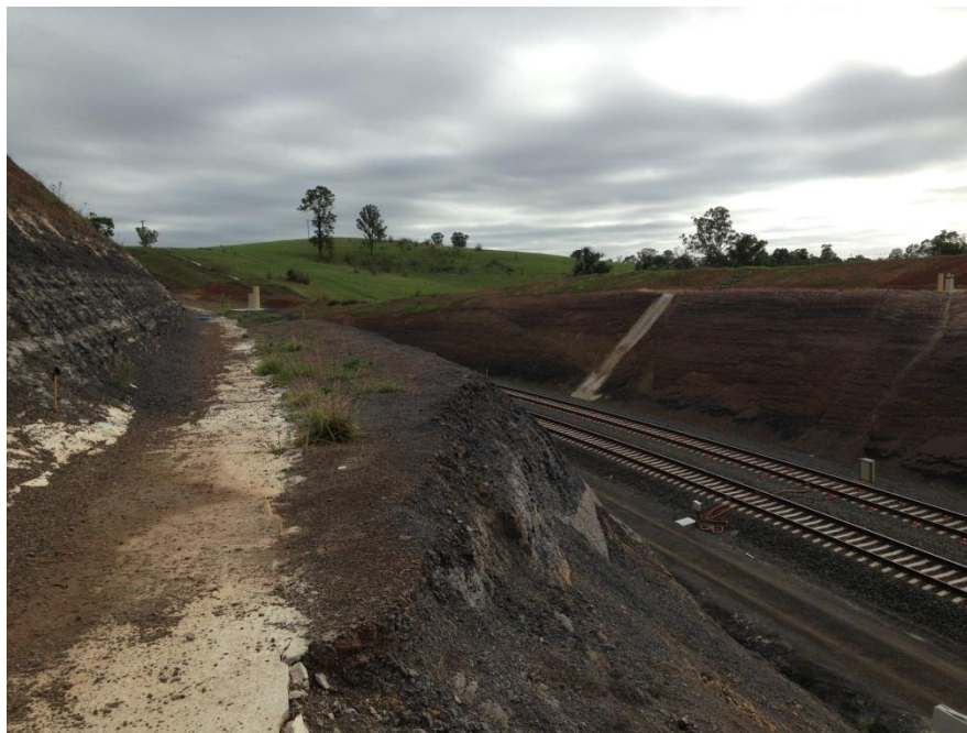
Fig. 2.6 Total Station 1 and 2 across the railway track
