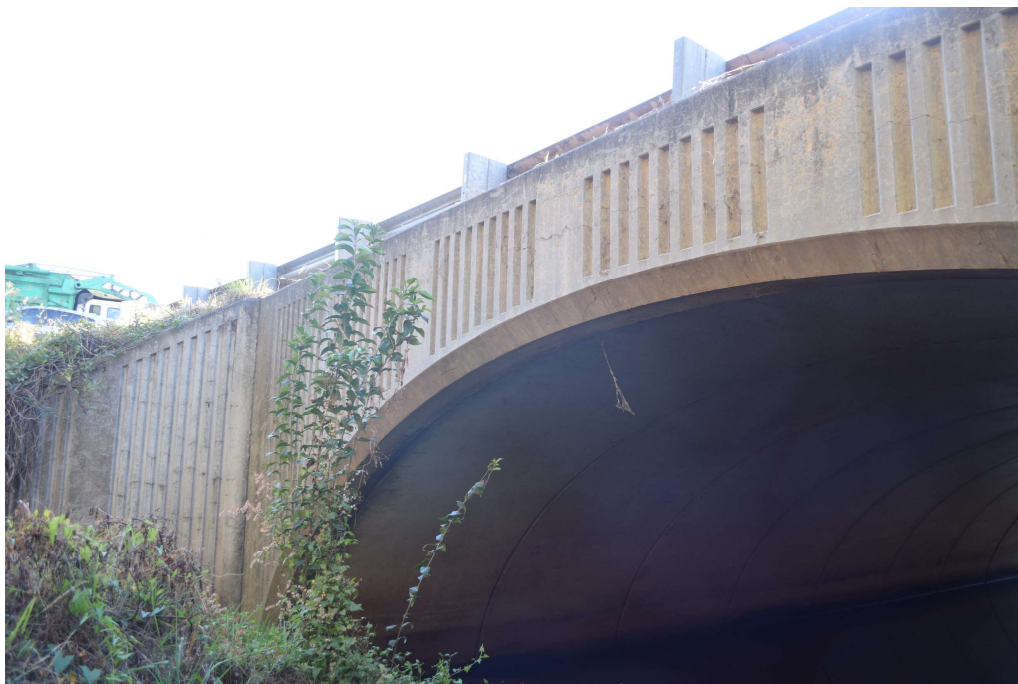
Figure 3 Northern end of western spandrel panel.
