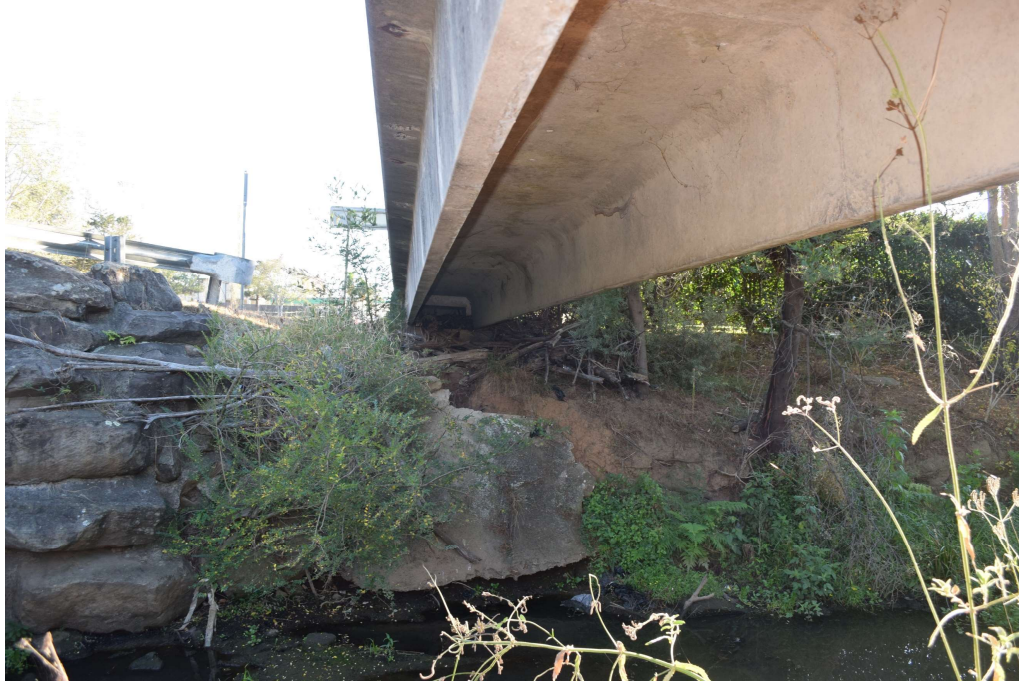
Figure 16 Precast concrete Double-T pedestrian bridge
