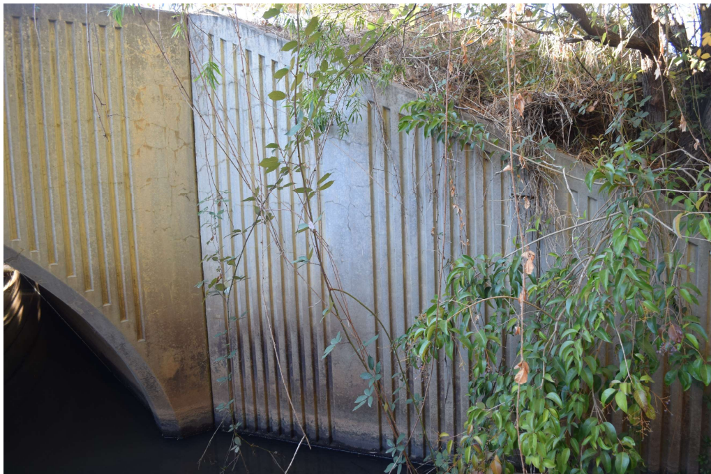
Figure 5 South-western precast concrete wingwall on Country abutment.
