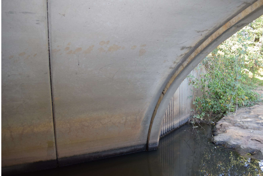
Figure 8 View of overlap of spandrel soffit and arch panels
