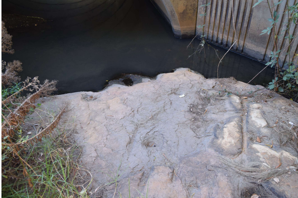
Figure 6 Sandstone rock bar upstream of the road bridge.
