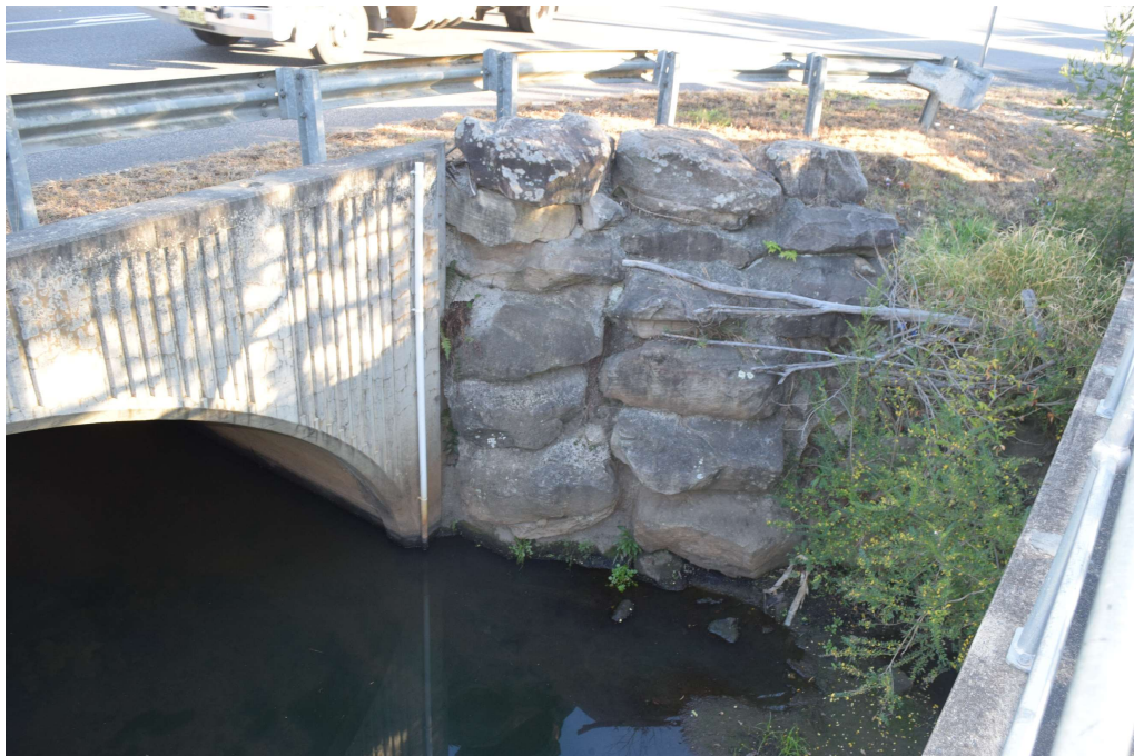
Figure 11 North-eastern riprap wingwall on the Sydney abutment.
