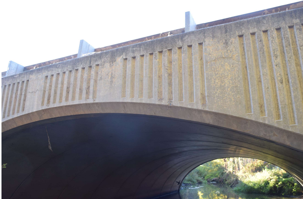
Figure 4 Spandrel midspan on western elevation.
