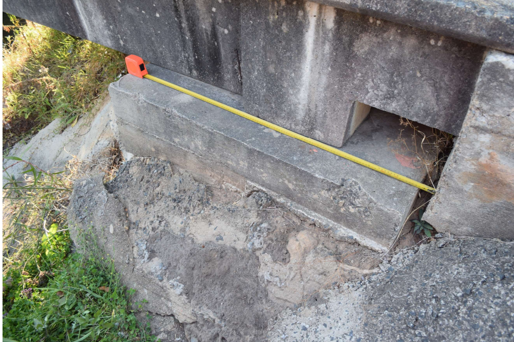
Figure 18 Southern abutment showing concrete shotcrete revetment.
