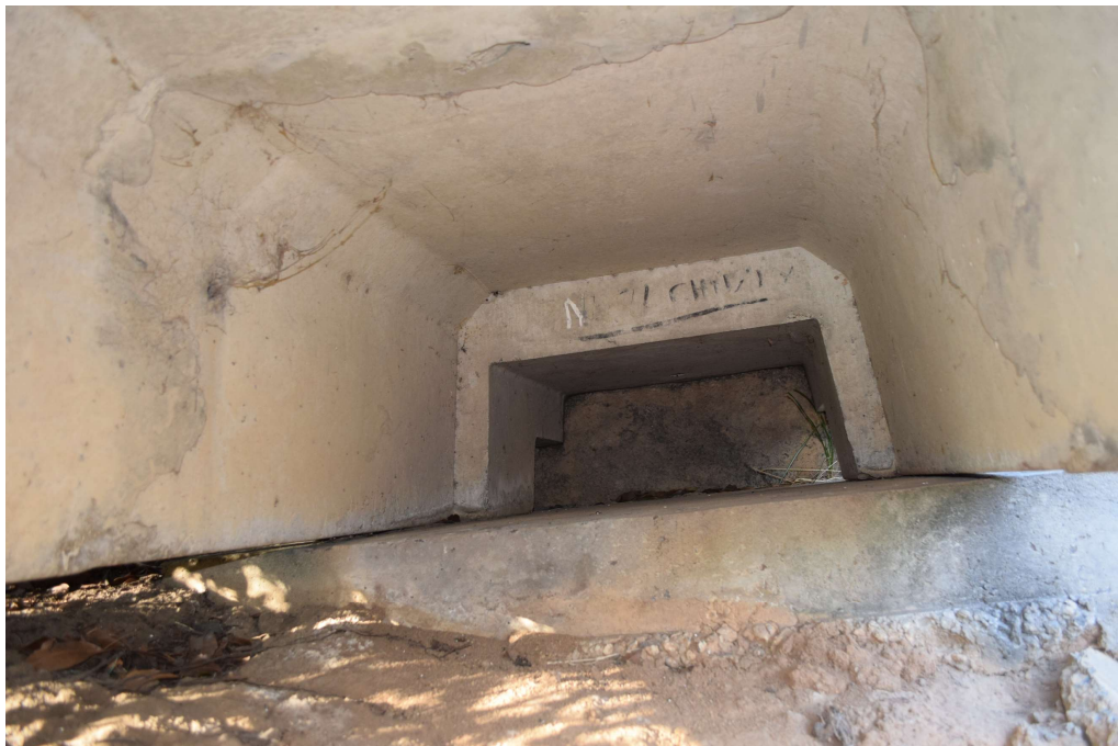
Figure 17 Southern abutment slab possibly founded on bored concrete piers
