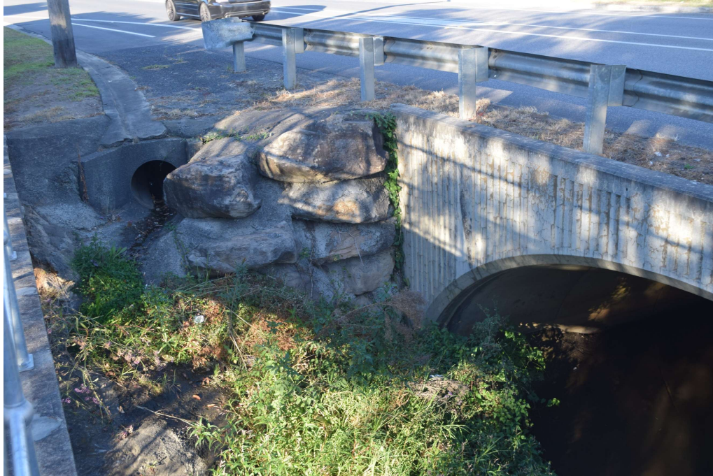
Figure 12 South-eastern riprap wingwall on the Country abutment.
