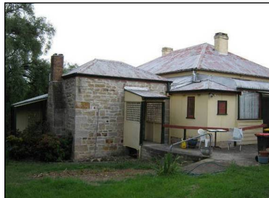
Plate 7: The south-east corner of the house, showing the stone building that was possibly the kitchen (source: Atkinson 2009).
