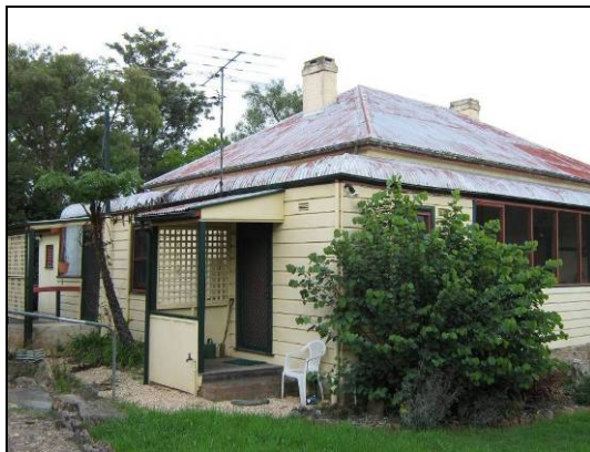
Plate 6: The north-east corner of the cottage (source: Atkinson 2009).
