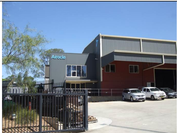
Figure 12 15 Redbank Place large structural steel portal frame with gantry crane and tilt-sensitive equipment. Two-storey tilt panel wall framed office
