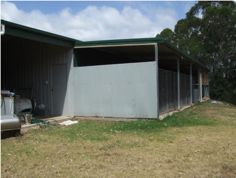
Figure 57 Steel framed shed
