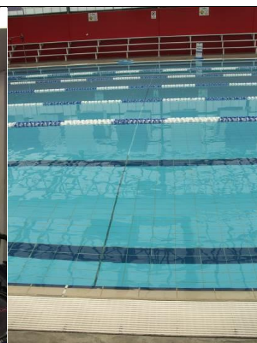
Figure 46 Indoor pool expansion joints
