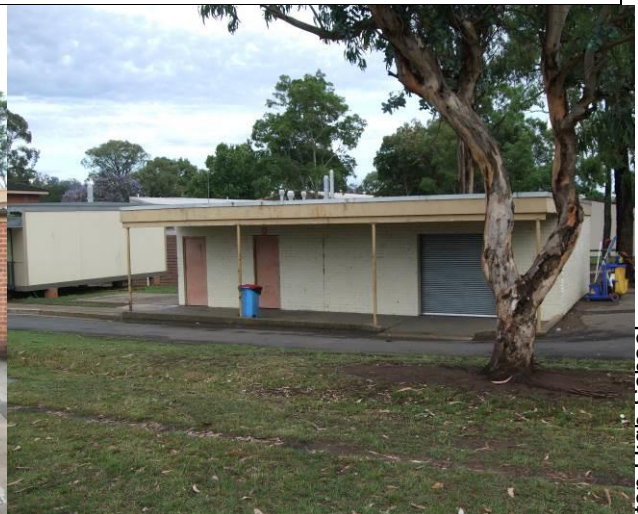
Figure 30 Articulated brick shed on a concrete ground slab PAR_210_pa33
