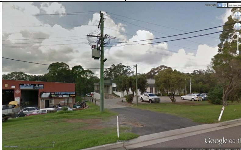
Figure 14 Single storey brick office at the front of a ductile structural steel portal framed structure at 61 Bridge Street on left hand side of image with the reinforced concrete framed SES building structure with cavity brick wall panels at 65 Bridge Street on right hand side of image
