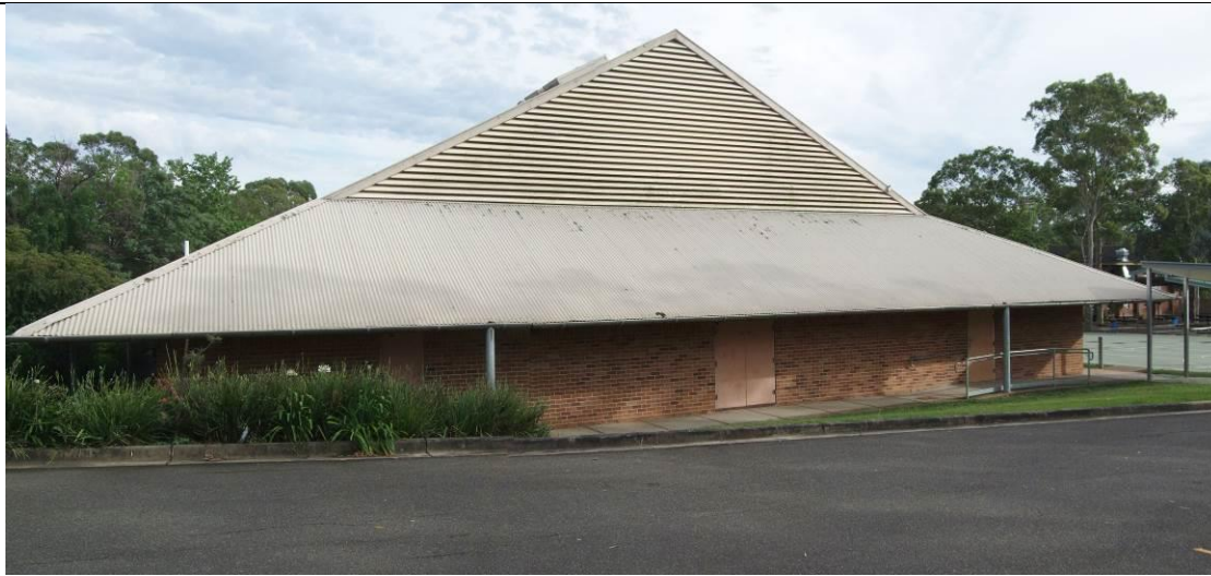
Figure 26 Multi-purpose hall PAR_210_pa16
