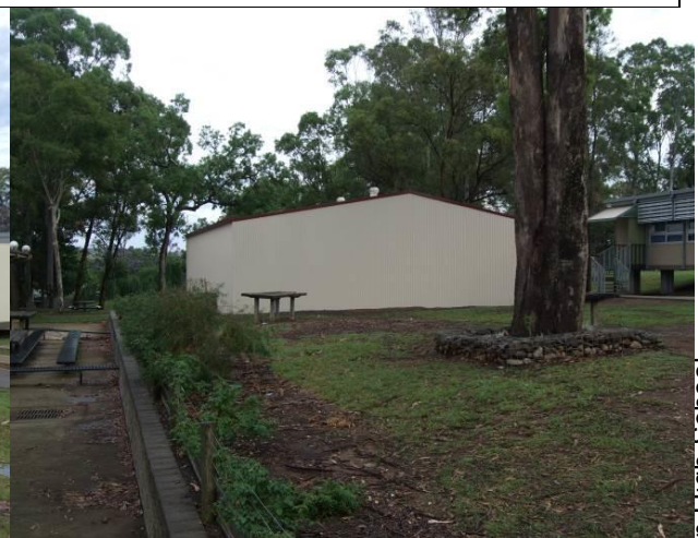
Figure 25 Ductile structural steel storage shed PAR_210_pa32
