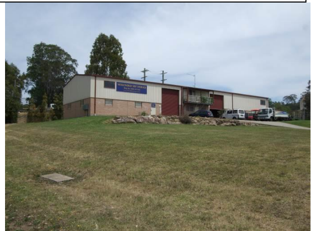
Figure 13 3 Redbank Place storage building with 2.4metre high articulated perimeter cavity brickwork and clad metal framed walls around a ductile steel portal framed structure
