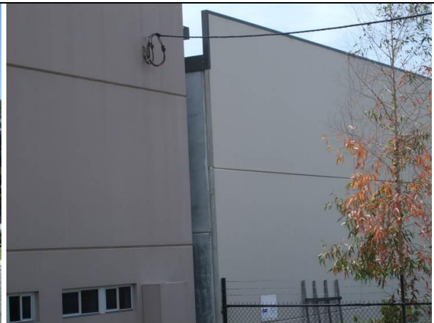
Figure 7 Interface between HH09/1a & 1b
