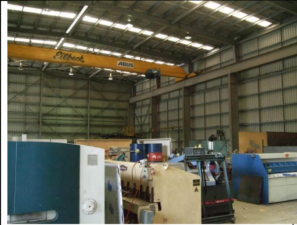
Figure 1 Internal photograph taken at 100 Bridge Street Picton, showing the steel portal frames, bracing panels, gantry crane and sensitive plant located on ground slab
