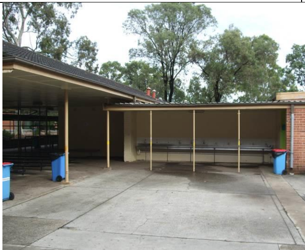
Figure 29 Canteen and amenities structures PAR_210_13 & 21 respectively
