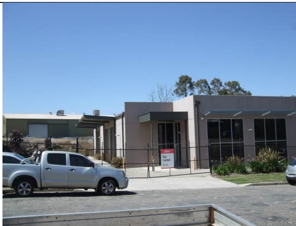
Figure 8 6 Redbank Place HH09/1a showing cantilevered steel awnings HH09/1c, 1d, 1e
