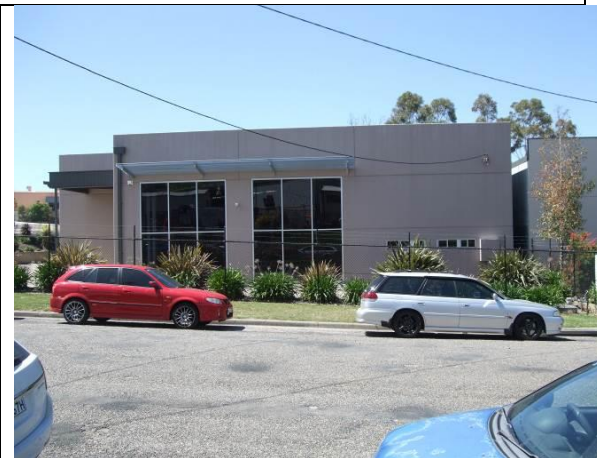
Figure 9 6 Redbank Place HH09/1a showing tilt panel walls
