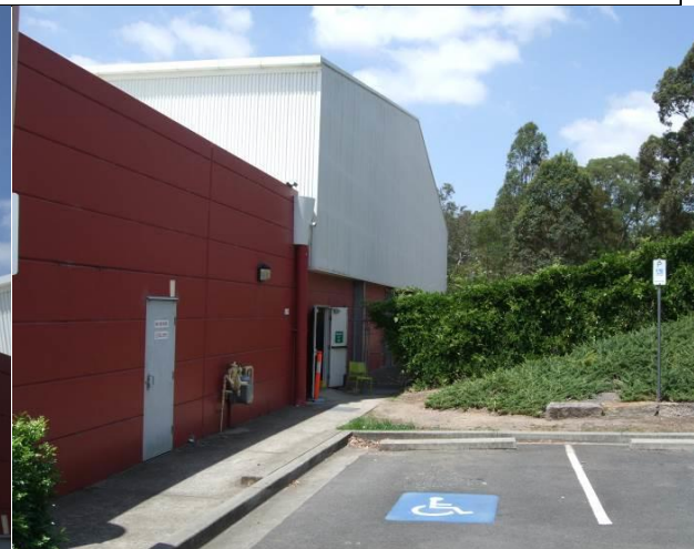
Figure 44 Southern wall to gymnasium & basketball courts
