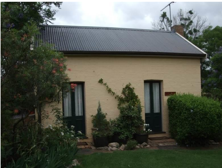
Figure 53 Northern elevation of the caretaker's cottage
