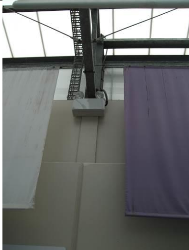
Figure 48 panel junction concealing steel portal frame column
