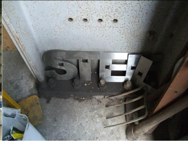
Figure 2 Steel portal frame baseplate hold-down bolts AT 100 Bridge Street
