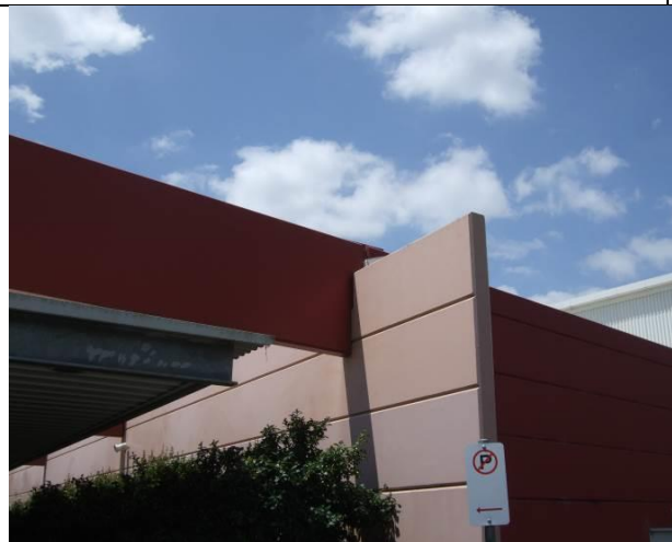
Figure 43 Structure over entry connecting with gymnasium
