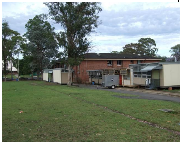
Figure 24 Demountable amenities blocks on left hand side PAR_210_pa53 & 54 and the GLA buildings on right hand side of the image PAR_210_pa 27 to 29.
