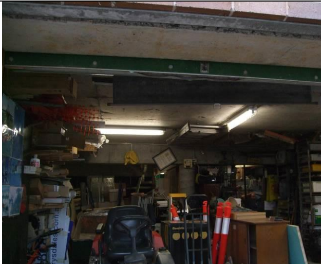
Figure 32 Block J PAR_210_pa12 under croft showing beam/slab and columns
