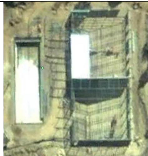
Figure 42 Olympic Pool and Main Building 2002
