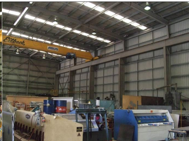
Figure 4 100 Bridge Street equipment
