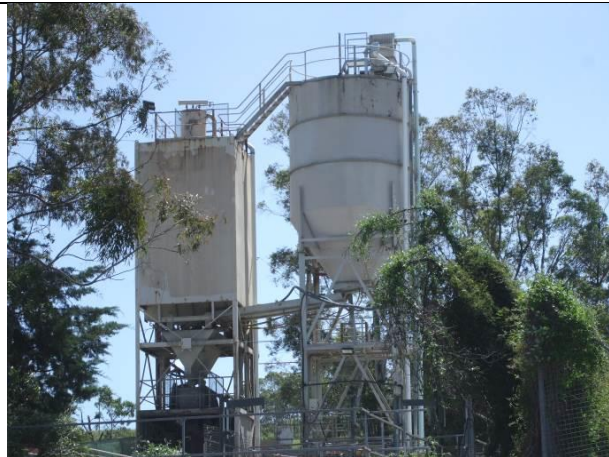
Figure 10 Hoppers HH07/2d and HH07/2e left and right respectively at 19 Redbank Place
