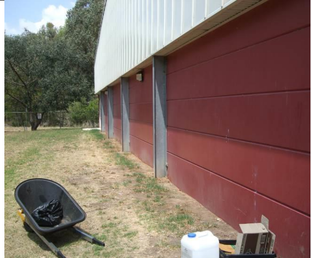
Figure 49 External view of north elevation wall looking south
