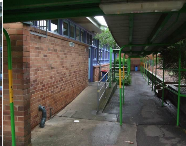
Figure 18 E Block looking south
